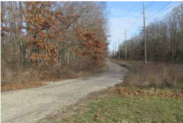
Existing access road to electrical substation
